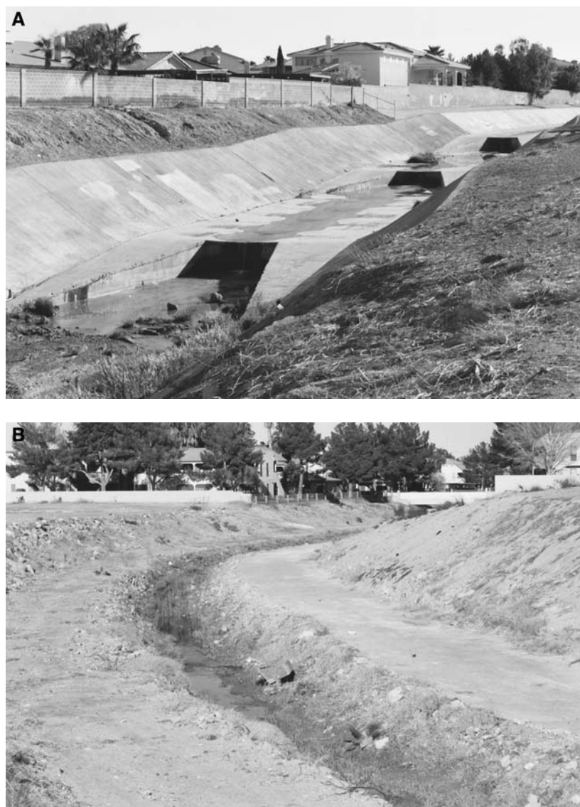
FIGURE 7.12 A modified wash in Las Vegas, NV: (A) a concrete-lined reach and (B) a downstream reach with a more natural two-stage geometry. (Courtesy John Lyon.)
