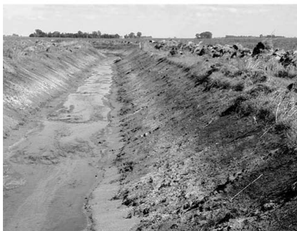
FIGURE 7.8 Large agricultural drainage ditch in Minnesota (A) before cleanout and (B) after cleanout. (Courtesy Gary Sands.)
