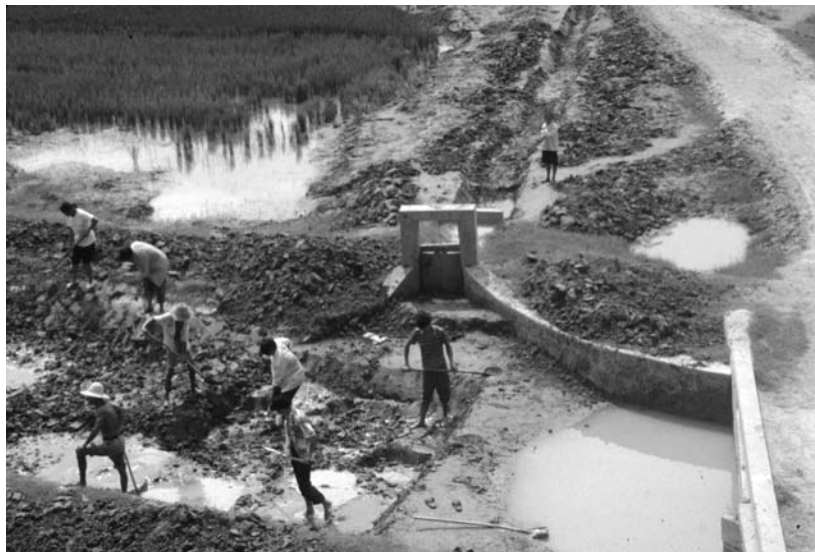
FIGURE 7.7 Cleaning out sediment in an irrigation channel in China.
