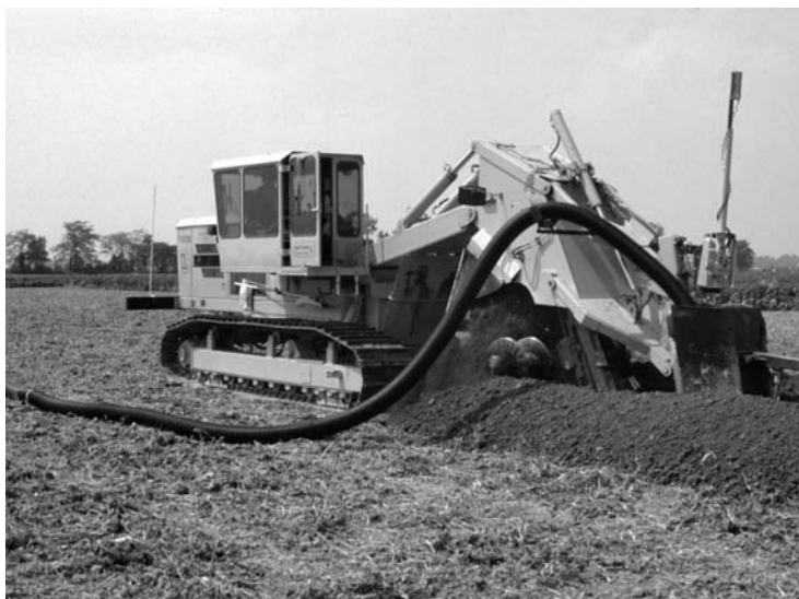
FIGURE 5.24 High-speed, and laser-controlled, installation of corrugated plastic drainage pipe.
