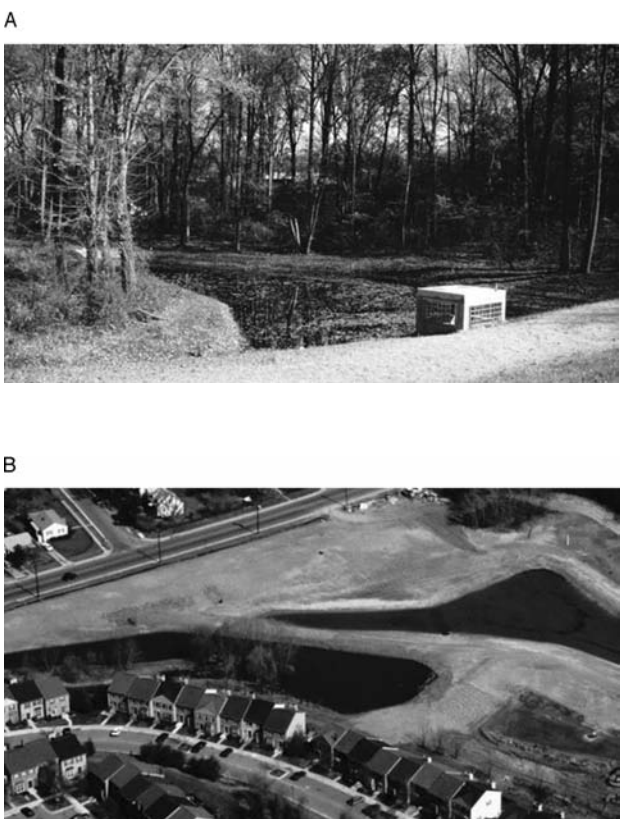
FIGURE 12.16 Urban detention basins: (A) small micropool extended detention pond; (B) multiple detention basins have improved water quality benefits. (Courtesy and copyright Center for Watershed Protection.)
