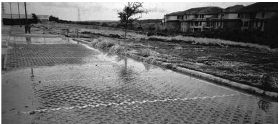
FIGURE 12.17 Pervious pavement shortly after a storm event shows increased runoff storage and then infiltration. (Courtesy and copyright Center for Watershed Protection.)
