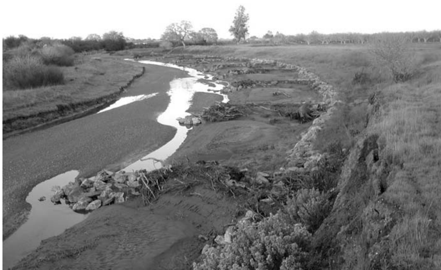
FIGURE 8.10 A bendway weir, Buckeye Creek, California, designed by John McCullah, Salix Applied Earthcare, and David Derrick, U.S. Corps of Engineers. (Courtesy and copyright Salix Applied Earthcare.)
