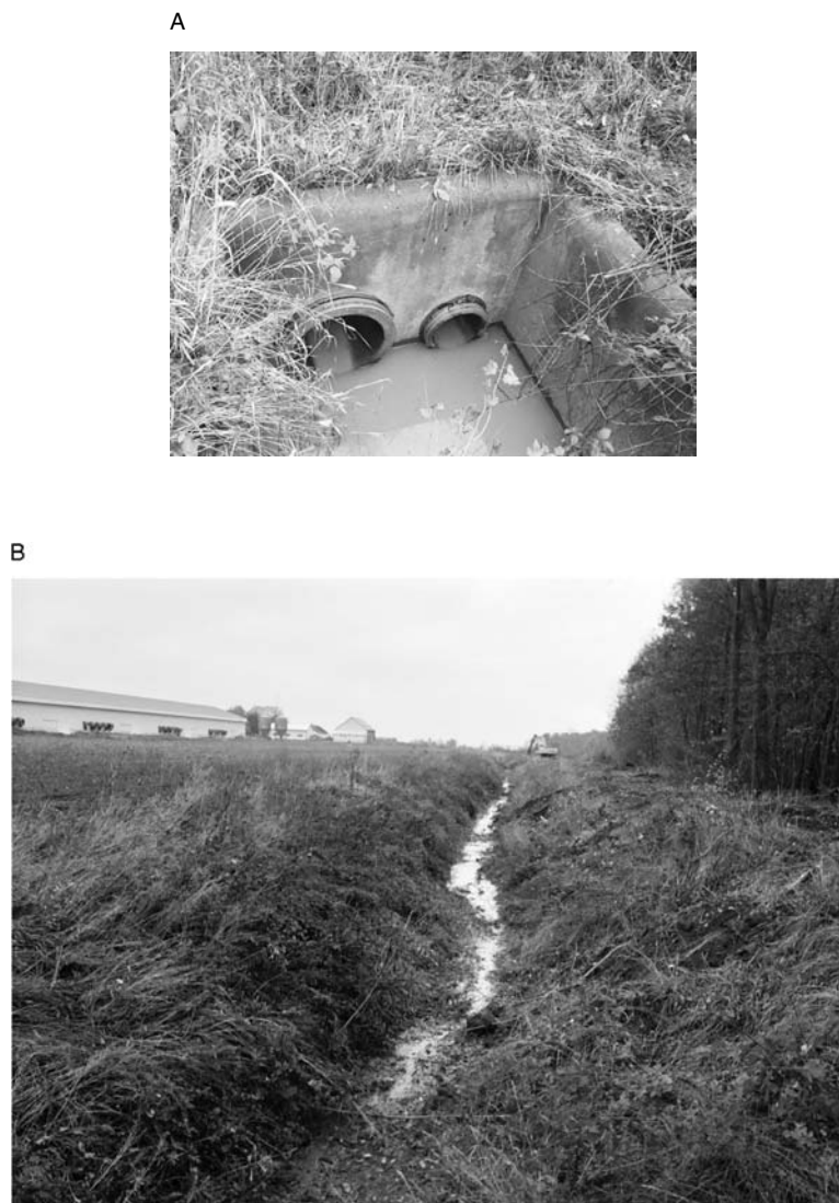
FIGURE 6.3 The Wabash River starts in Darke County, Ohio, as (A) outlets of two subsurface drainage mains and (B) a small drainage ditch.
